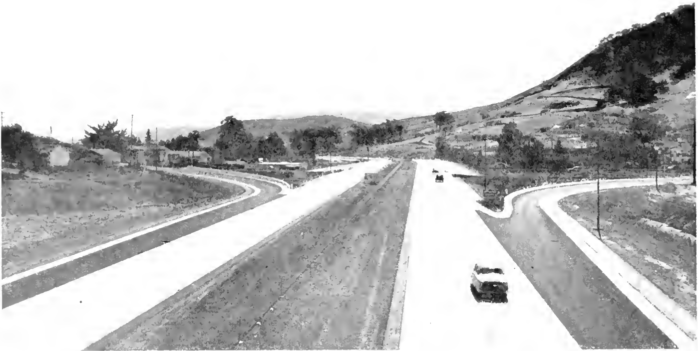
Looking south from Santo Roso Street overpass, showing on and off ramps from business district of San Luis Obispo
